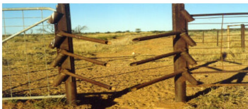
Figure 2: TGM cattle/sheep/goat trapgate – gravity operated spear design.
